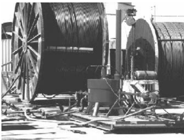
Cable Installation Operation
